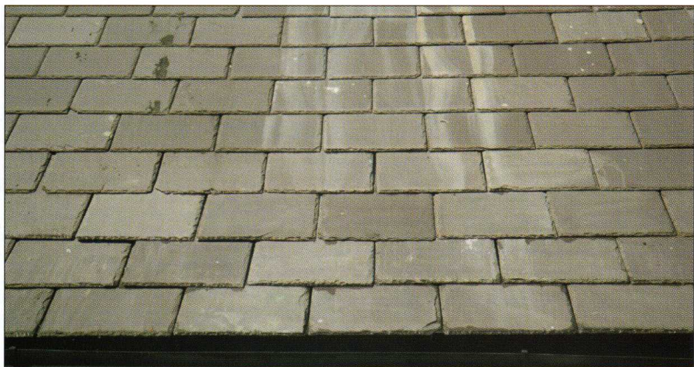
Repairs carried-out with 'Jenny Twin' system.
